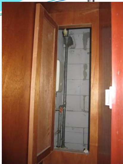
管槽 (Pipe duct)
