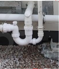
Replenishment of Sealing-trap
